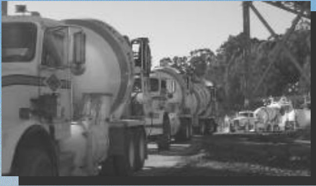
Trucks on way to placement site from SF cement plant.
