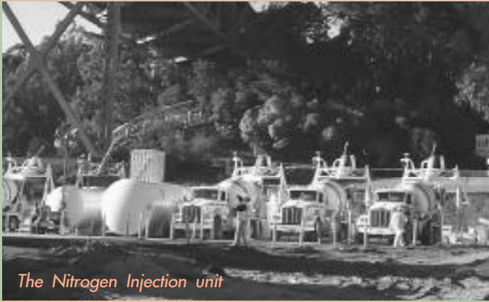
Nitrogen being shot into truck at jobsite
