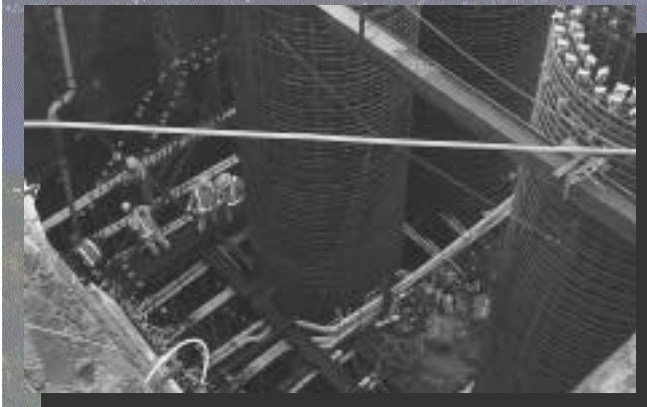
A view of workers down in the footings.
