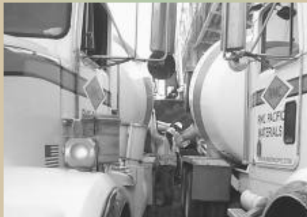
Space was sometimes scarce as multiple trucks navigate the huge job.
