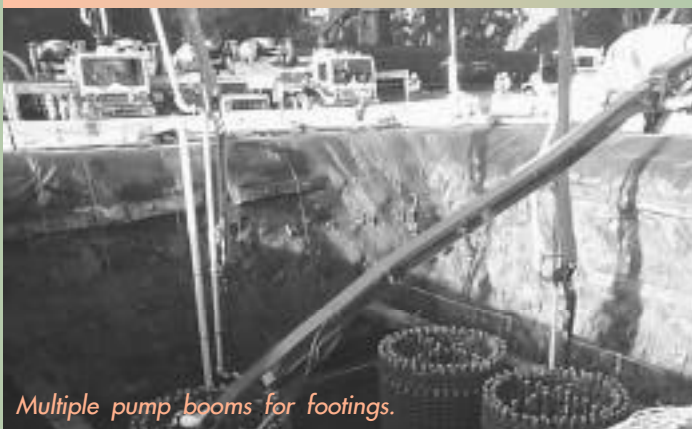
Concrete being placed in the footing
